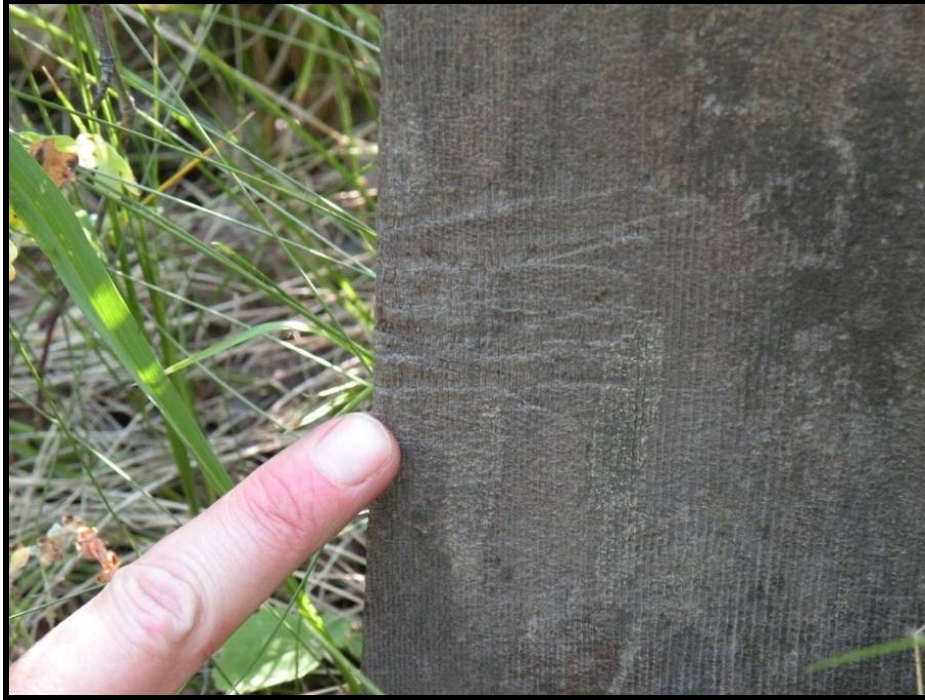
Figure 36. Damage on the edge of a wooden marker caused by a weed trimmer.
