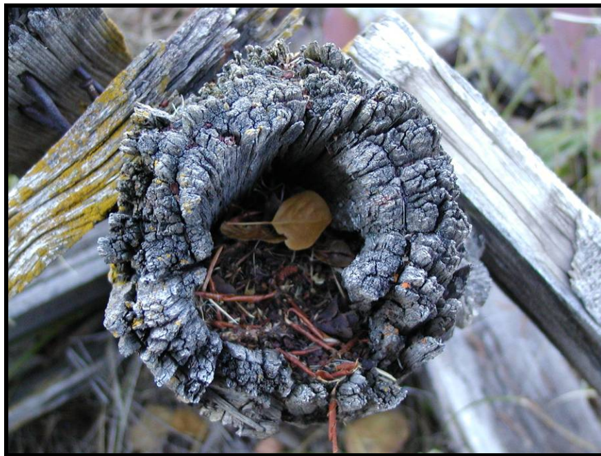
Figure 6. A grave enclosure corner post with debris collecting in a deteriorated area. This is an example of weathering that can lead to cavities susceptible to decay.
