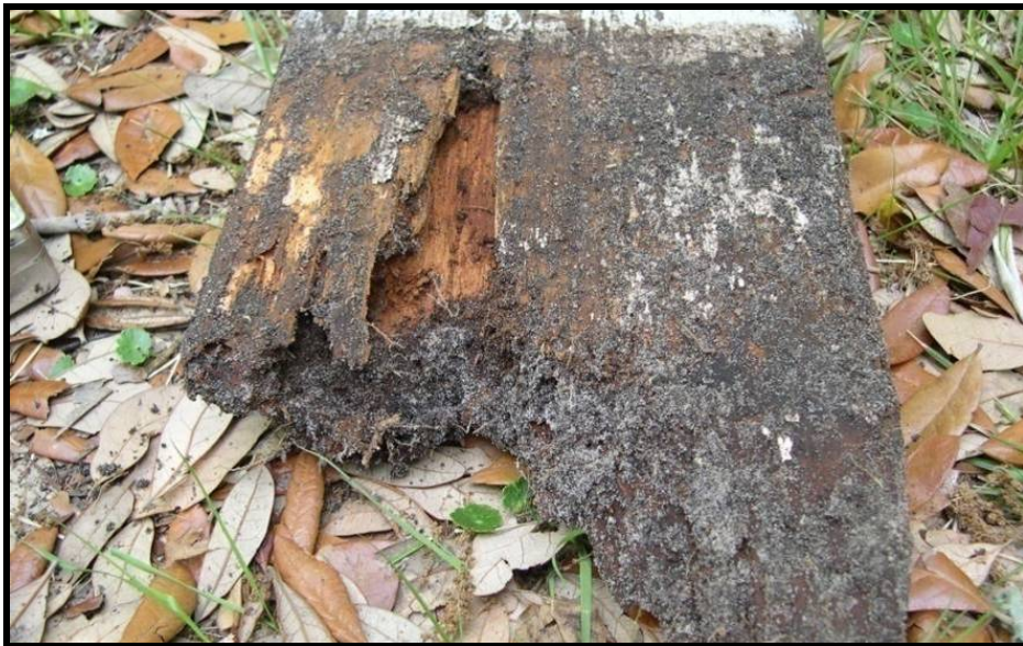
Figure 24. Loss of wood in the underground portion of a grave marker by subterranean termites.
