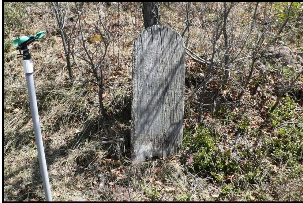
Figure 41. A water sprinkler located directly next to a wooden marker that is showing signs of decay at the base.
