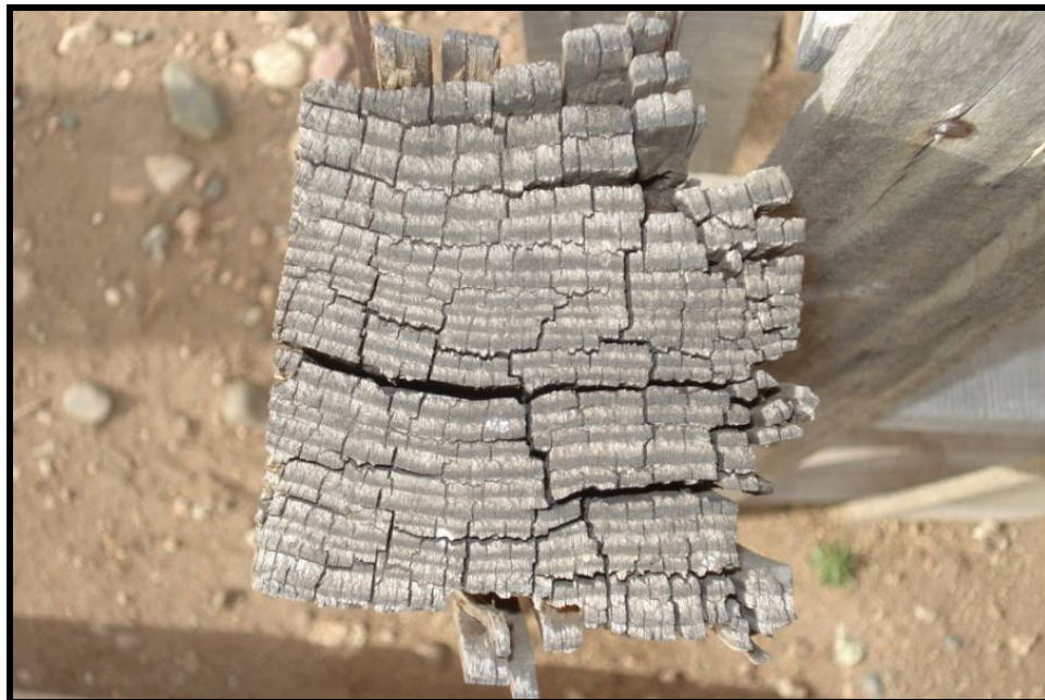
Figure 2. The top of a grave enclosure corner post showing splits developing from cyclic moisture or freeze/thaw episodes.
