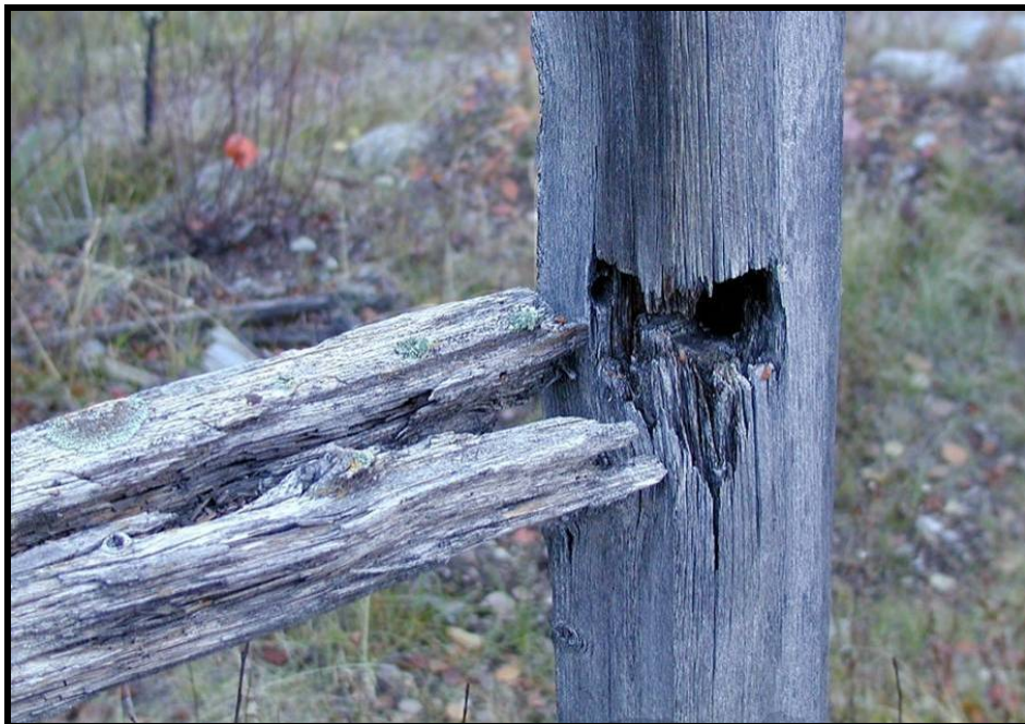
Figure 20. A grave enclosure corner post with signs of advanced internal decay and failure of a cross-member.
