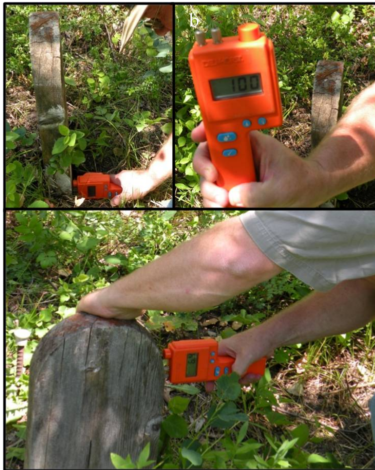
Figure 40. Taking moisture readings on a grave marker using a resistance-type meter. Image (a) shows a reading being taken at the base of the marker; (b) shows the digital readout of 10 percent; (c) shows another reading being taken at the top of the marker (where the moisture content reads 6 percent).
