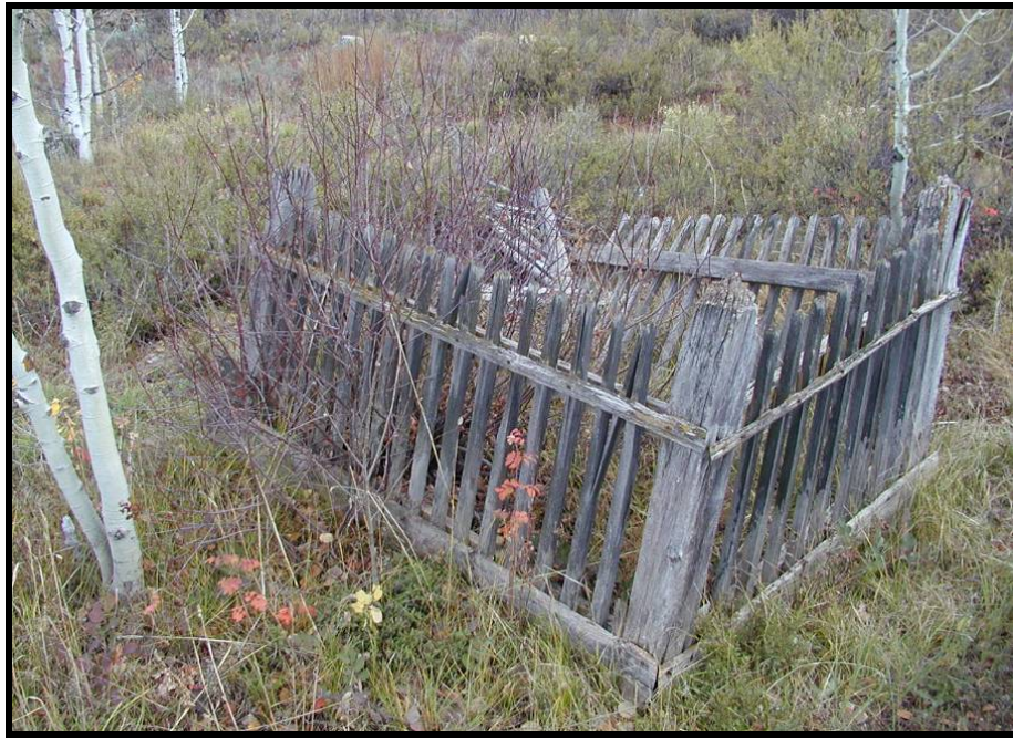
Figure 19. A grave enclosure in partial collapse due, in part, to decay of the corner posts at ground level.
