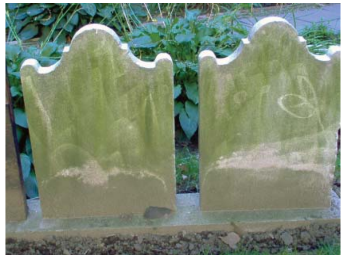
Figure 14. High-pressure water washing can damage grave markers. The photograph shows "wand marks" on the headstones produced by inappropriate pressure washing. Photo: Jason Church.
