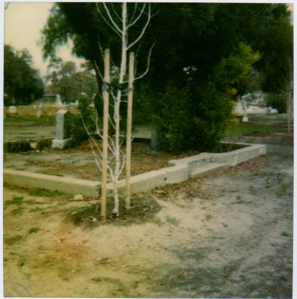
ELVYN PLOT. Near Woodside Rd. Tree planted too close to family plot boundary berm.
