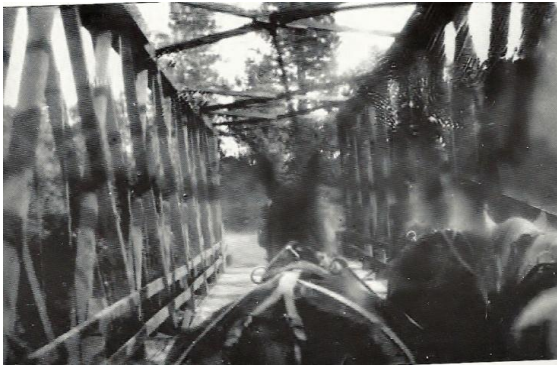
Hallidie's wire rope suspension bridge over Deer Creek in Nevada, with the first horses and cart crossing it in 1862. (A very old and fuzzy picture.)
