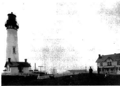
Pigeon Point Lighthouse, the Victorian keeper's house and the ramp.
