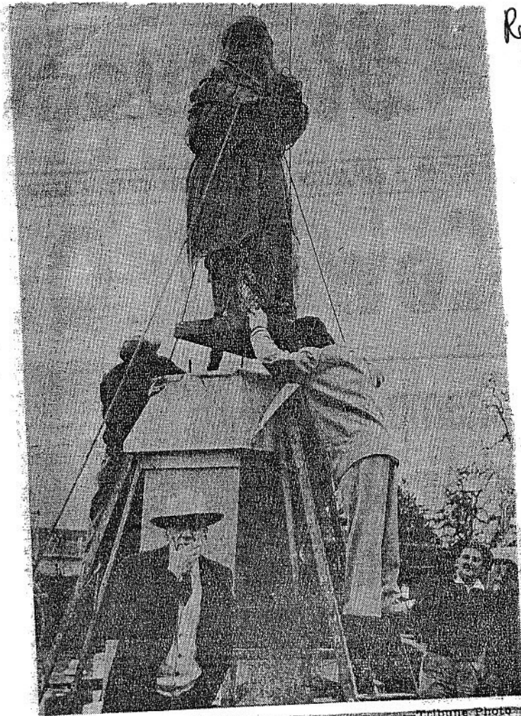
REPLACING CIVIL WAR MONUMENT HERE ... Ole Olson (left) Floyd Granger, center, and Pasco Balzarini, on ladder
